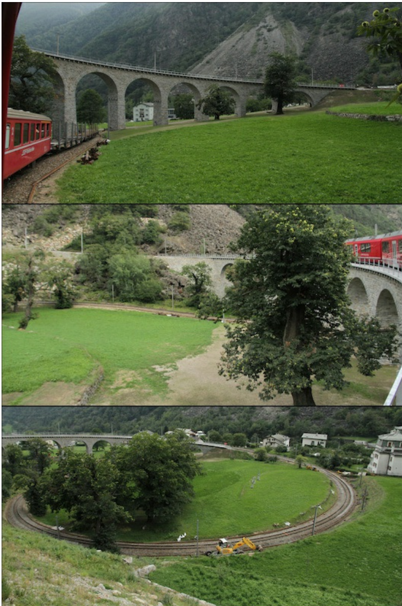
Those Swiss! Engineered spiral rail bridges on the Rhaetische Bahn.
